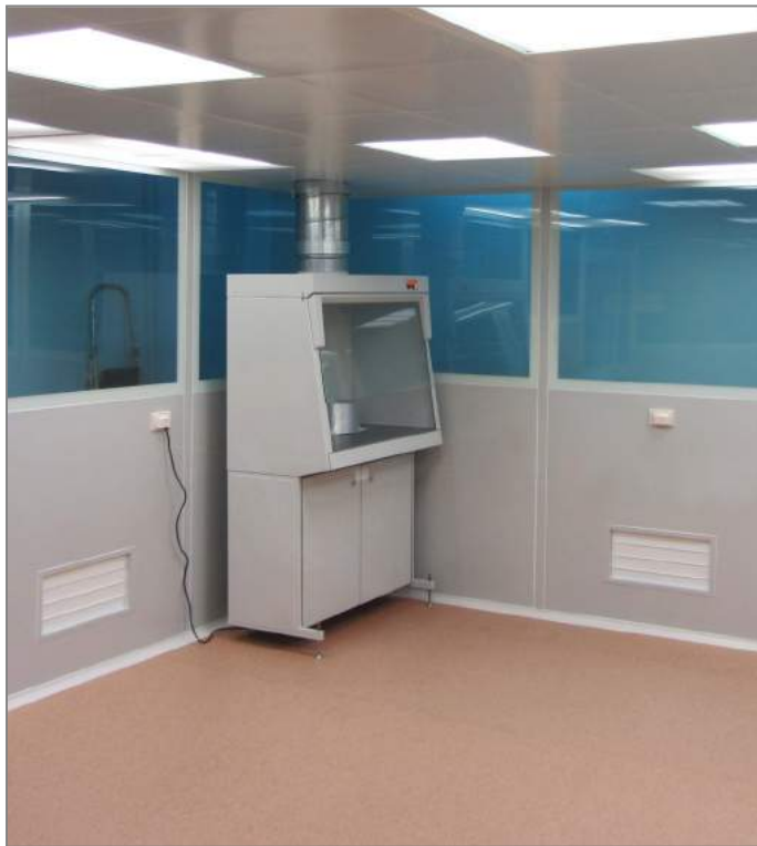
A fume hood in the clean zone Cleanliness class 7 ISO 14644-1 Assembly overall dimensions (LxWxH, mm): 4910x4310x2515
