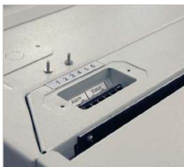
The cabinet is equipped with two voltage free outputs for connecting external devices for the purpose of transmitting information about the current and operation status of the cabinet.
